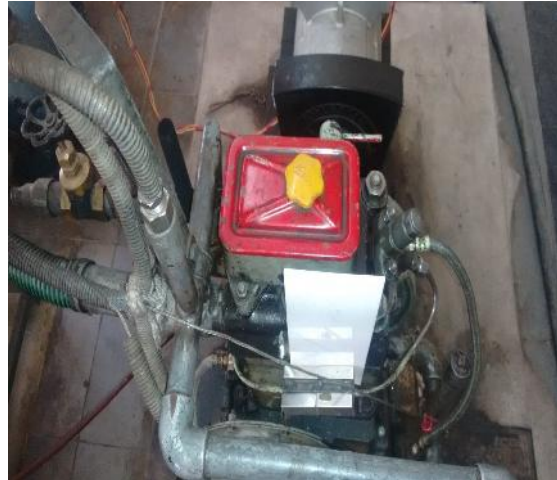
Figure- 3 Installation of Magnetizer Set Up on the fuel line.
